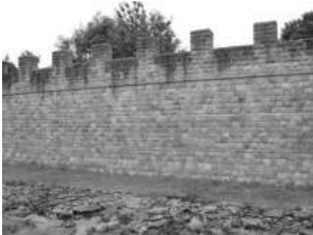
Figure 9. Reconstruction of stone curtain of Hadrian's Wall at Wallsend, with original Roman foundations in foreground. (Photo: author)
