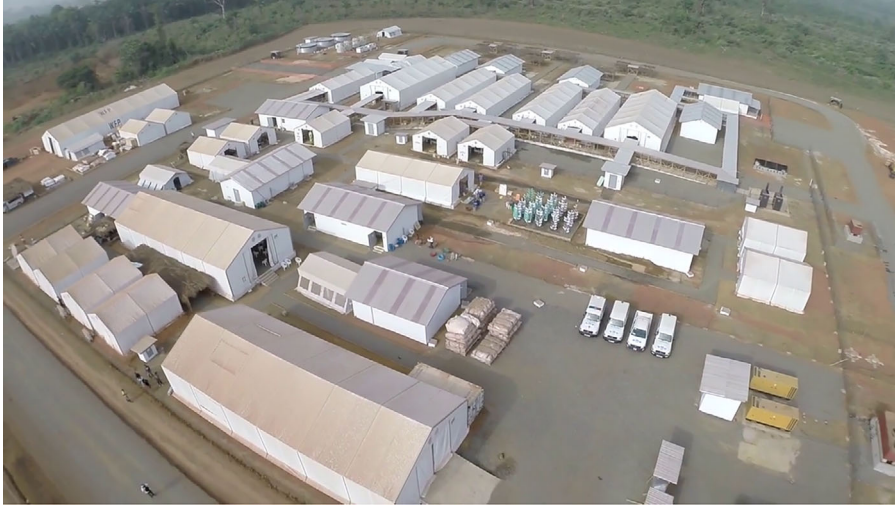
Figure 1. Aerial photograph of Moyamba ETU. Reproduced with permission. (Credit: The Royal Engineers.)
